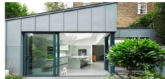
zinc roofing / upper level walling
