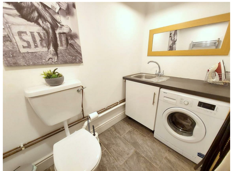
Fitted with a base unit with worksurface over, sink unit with mixer tap, plumbing for washing machine, w/c and heated towel rail.
