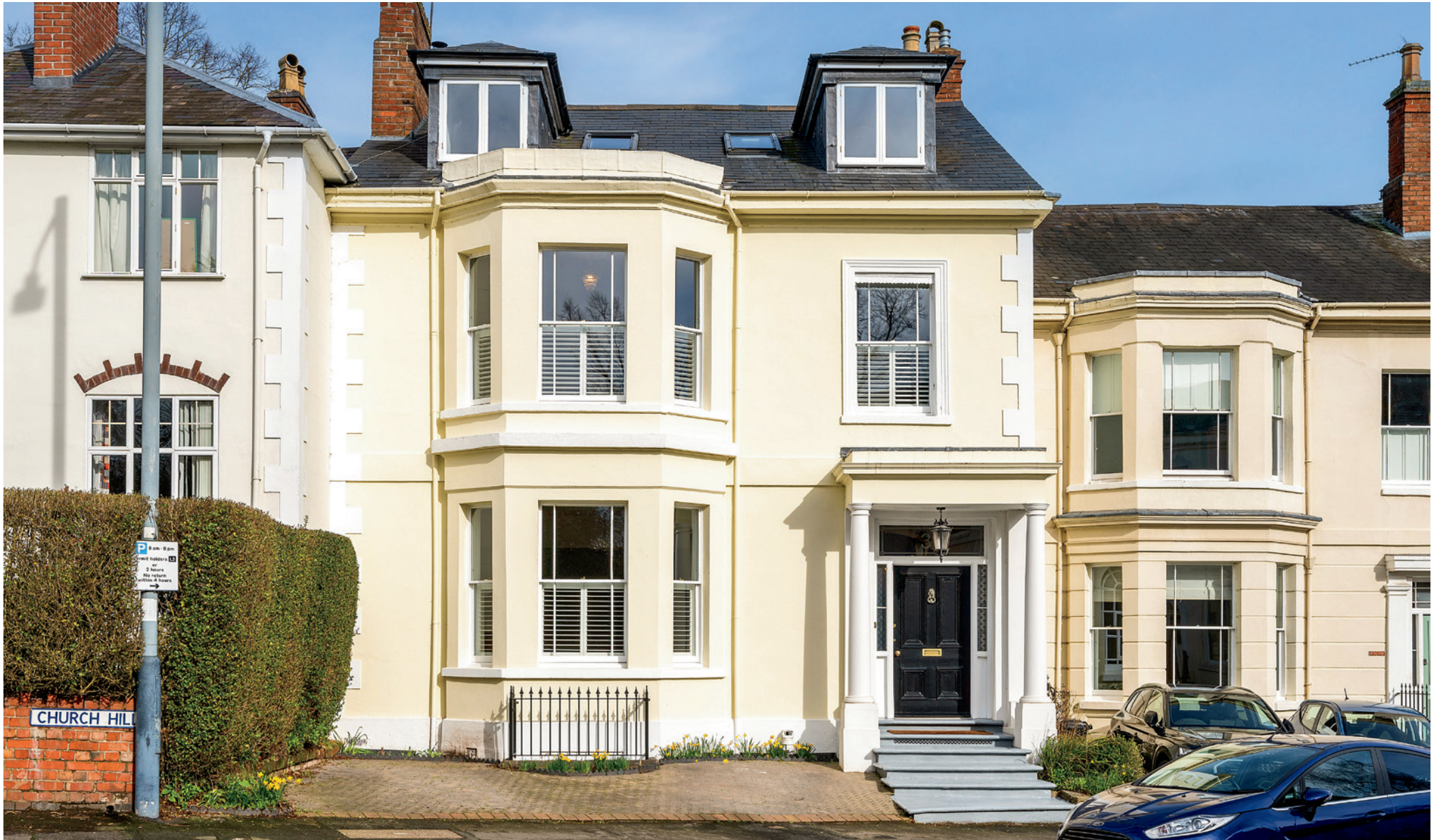
Melbourne Villa Church Hill | Leamington Spa | CV32 5AY
