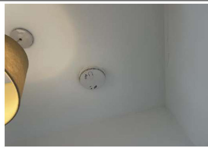
Location – Hallway Ceiling
