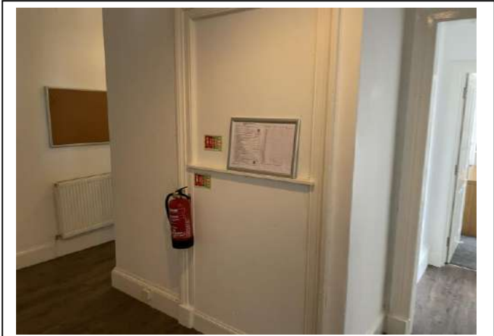
Location – Hallway Wall
