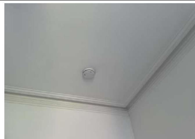
Location – Bedroom Ceiling
