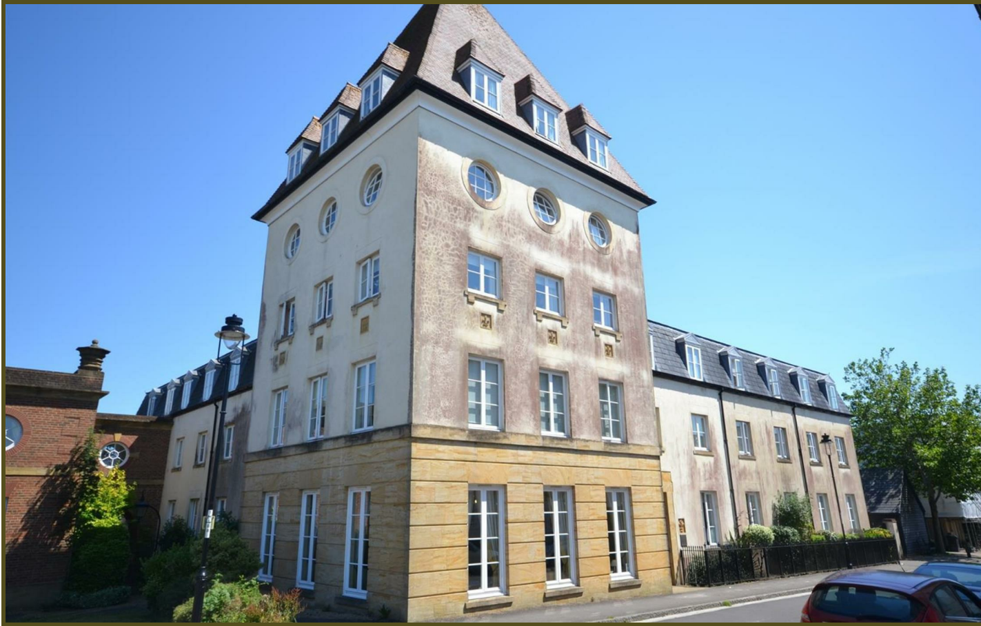
Middlemarsh Street, Poundbury
