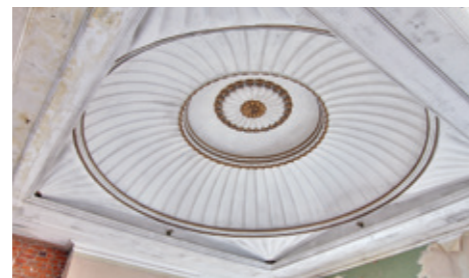
Existing domed roof
