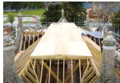
New timber roof
