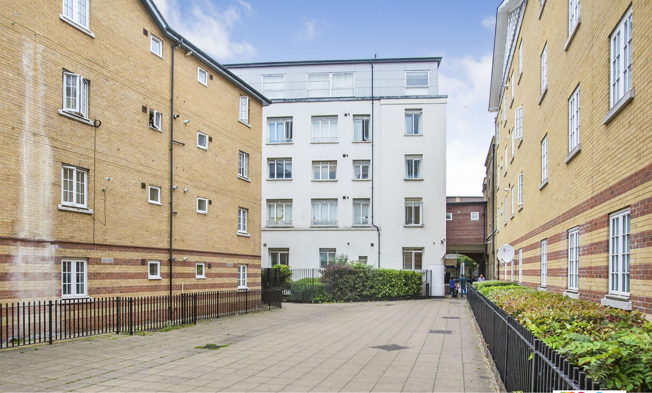
The Gatehouse High Street, Romford RM1 1AN
