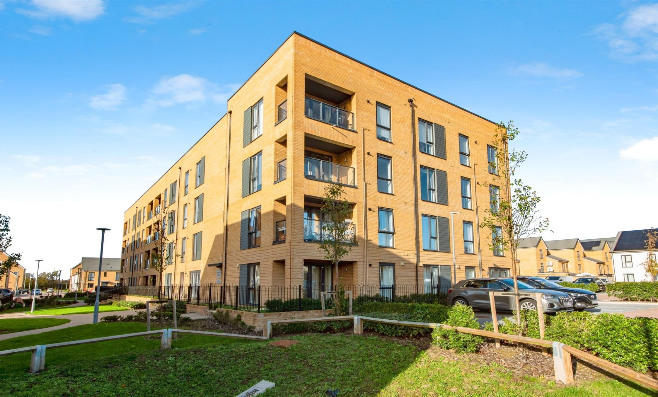
Ambrose Court, Windstar Drive, South Ockendon RM15 5LF
