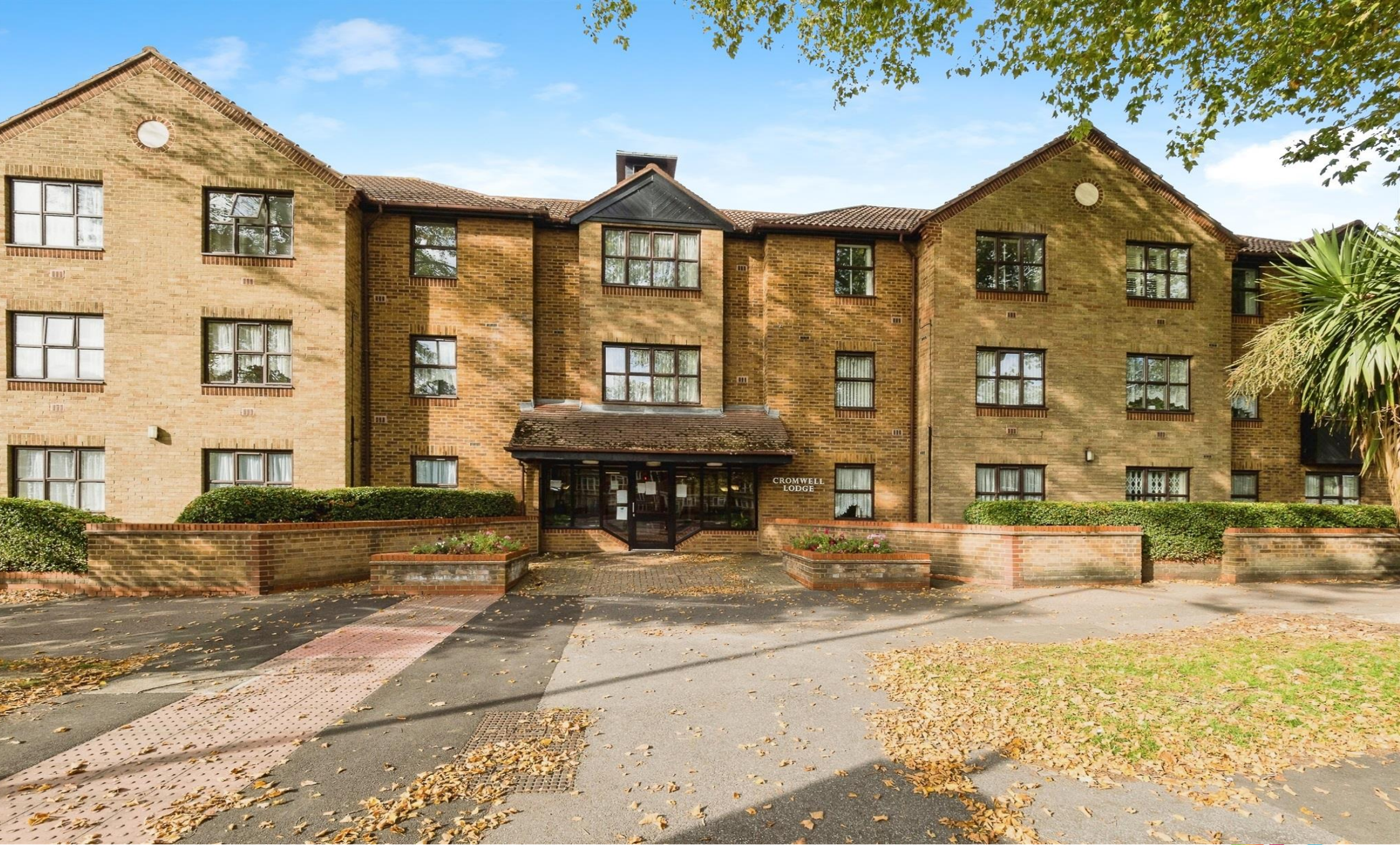
Cromwell Lodge, Longbridge Road, Barking, IG11 8UB
