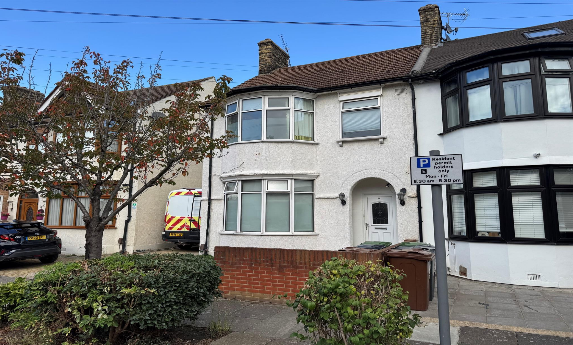
Netherfield Gardens, Barking, IG11 9TN
