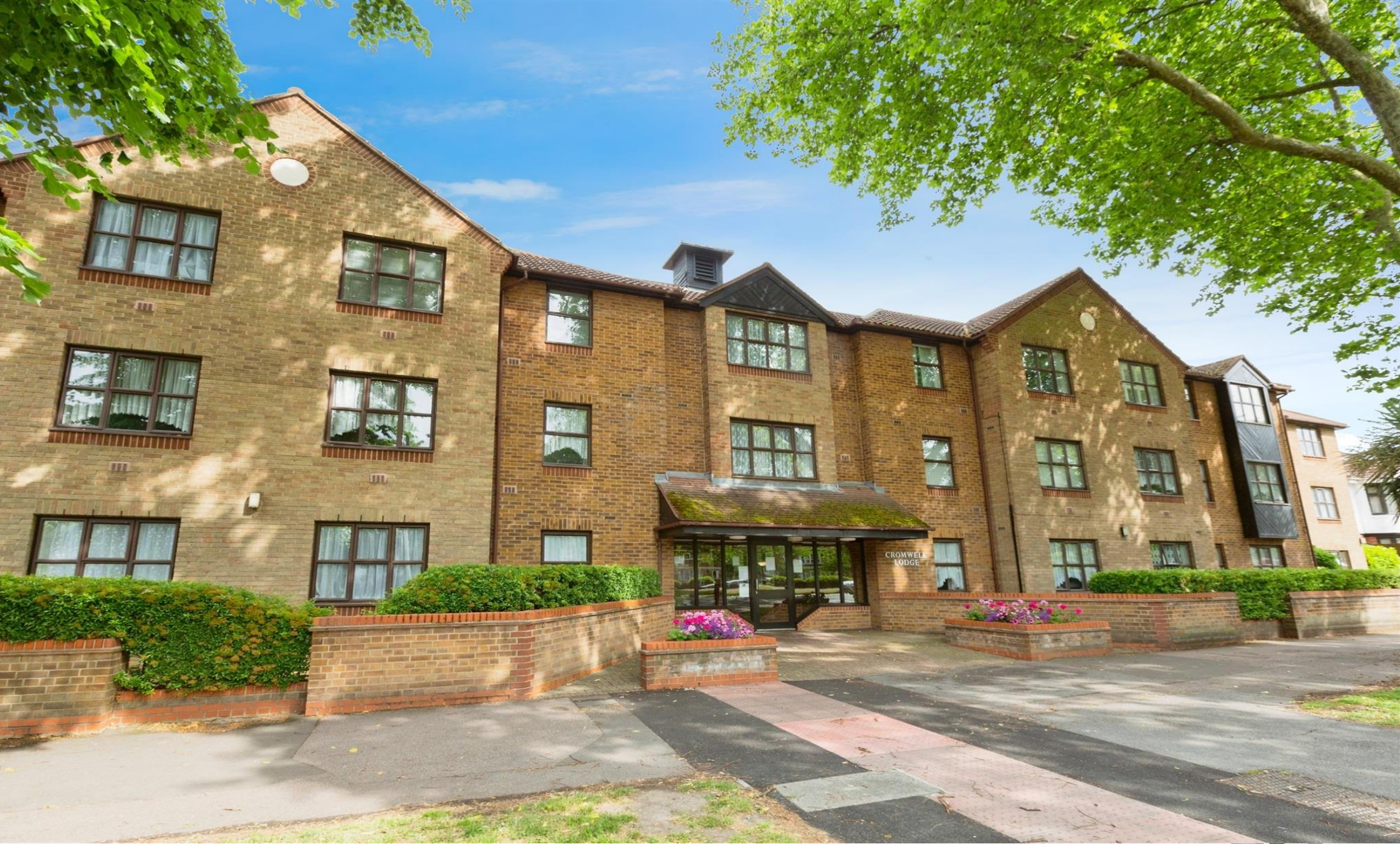
Cromwell Lodge, Longbridge Road, Barking, IG11 8UB
