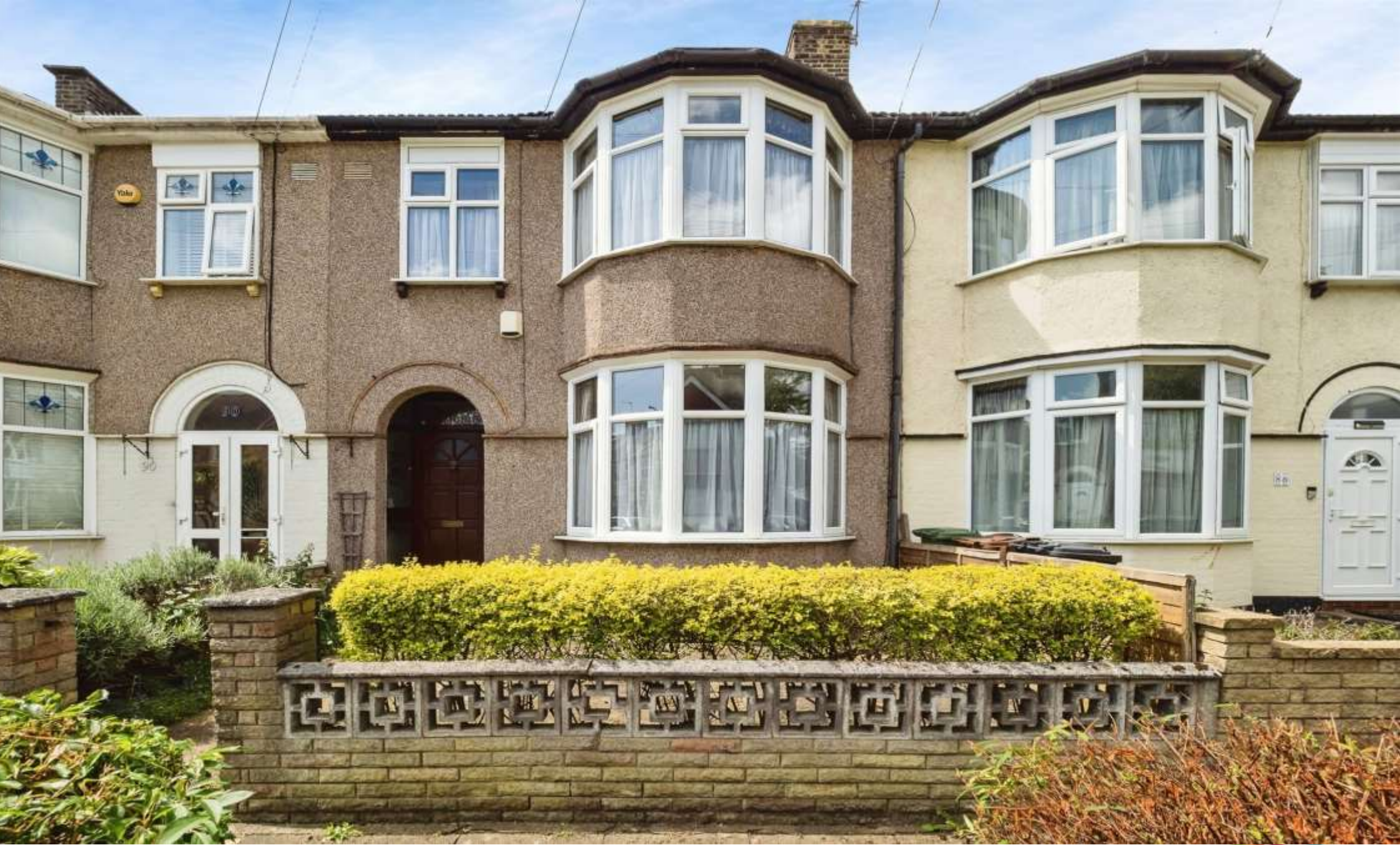
Netherfield Gardens, Barking, IG11 9TN
