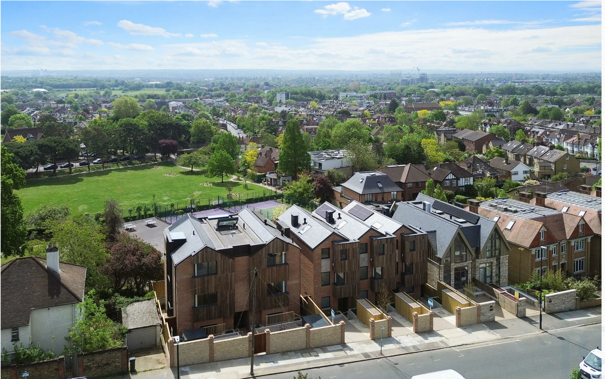
Cottenham Park Road, Wimbledon, SW20 0SB
