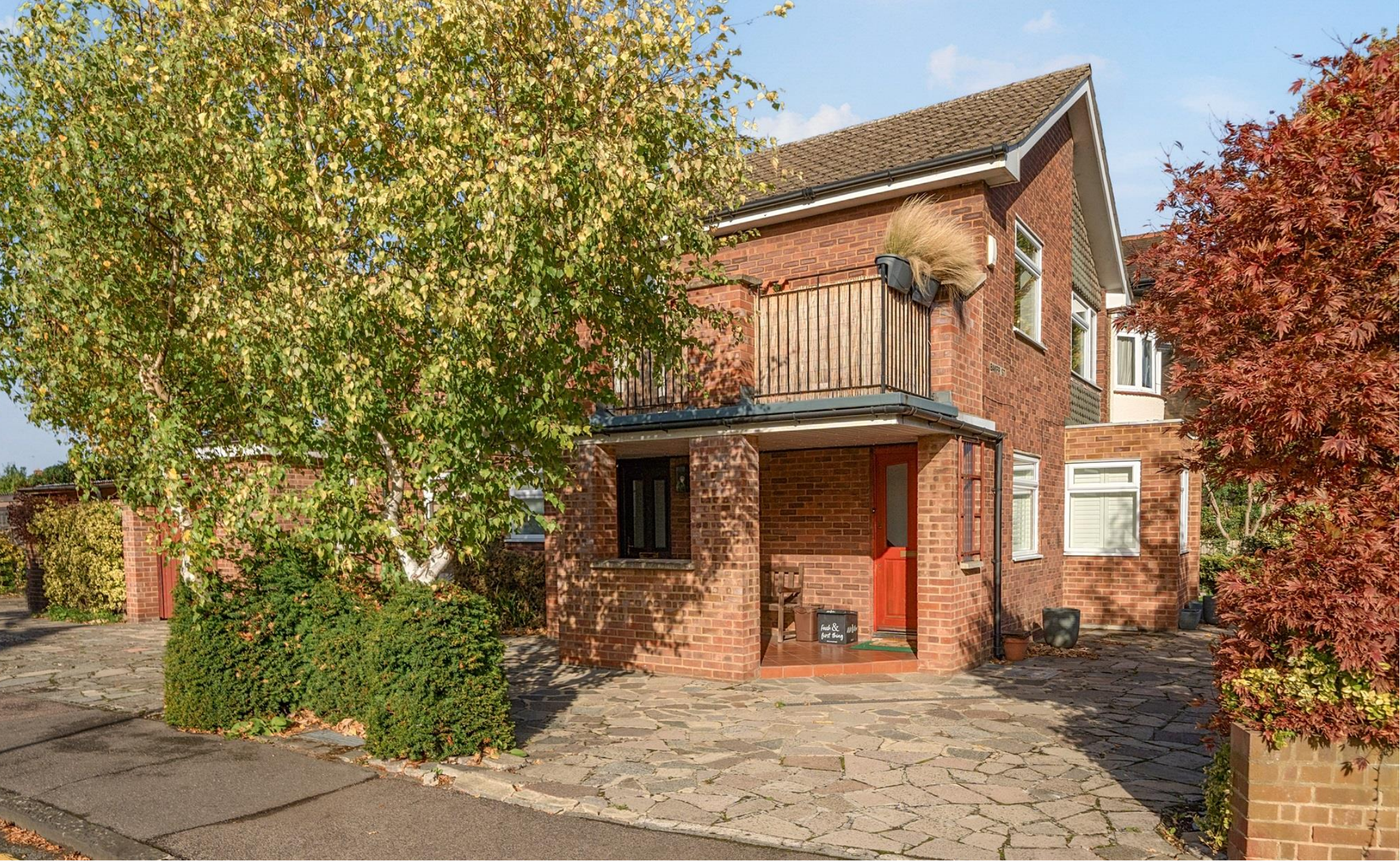
Baker Street, Enfield, EN1 3JS
