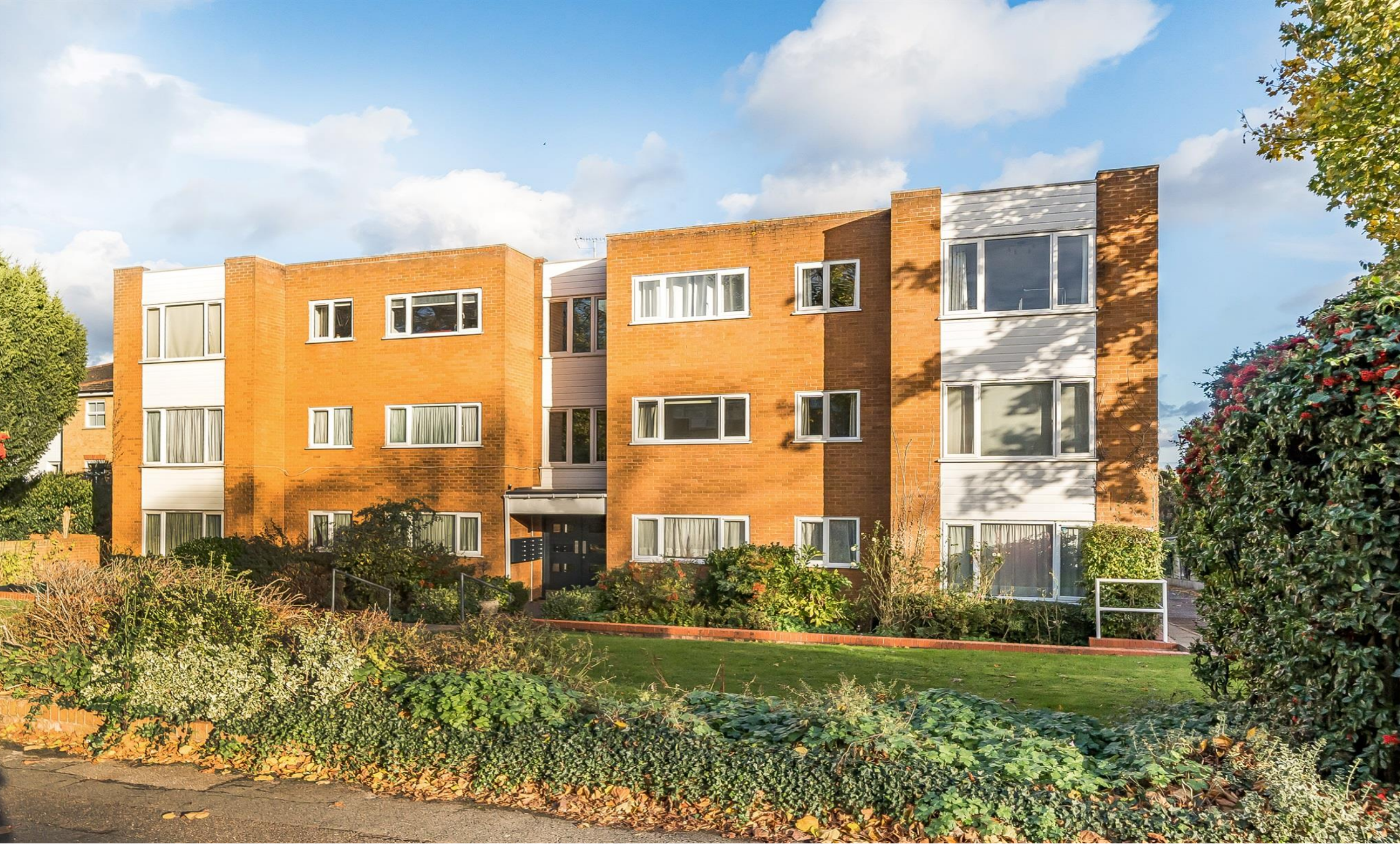
Butterfield House, Bycullah Road, Enfield, EN2 8EZ
