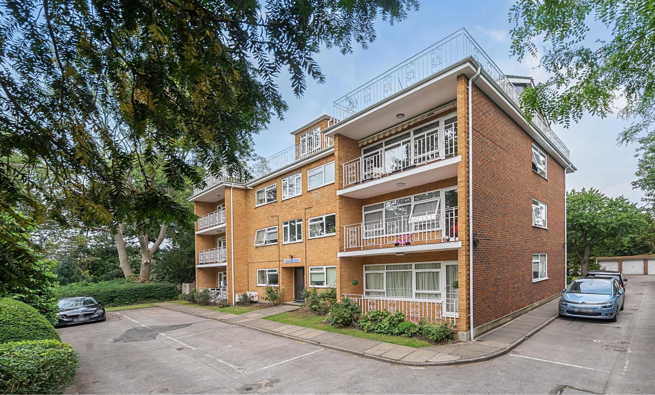
Halcyon House, Private Road, Enfield, EN1 2EJ
