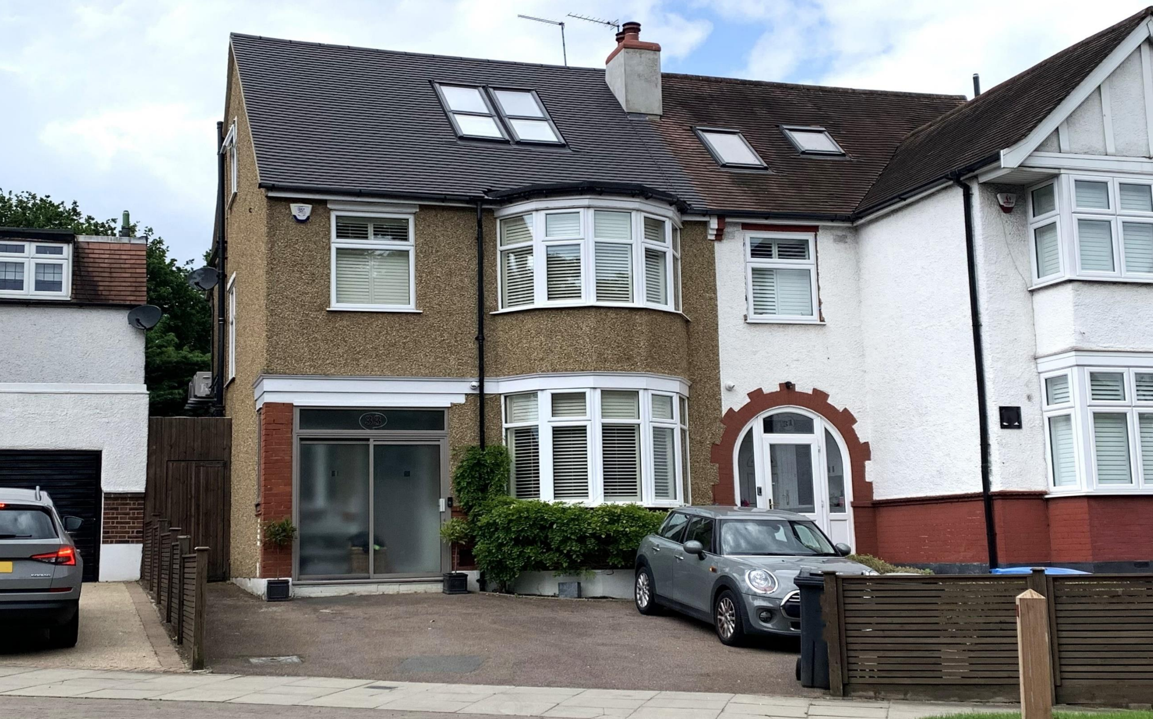
Old Park Avenue, Enfield, EN2 6PJ
