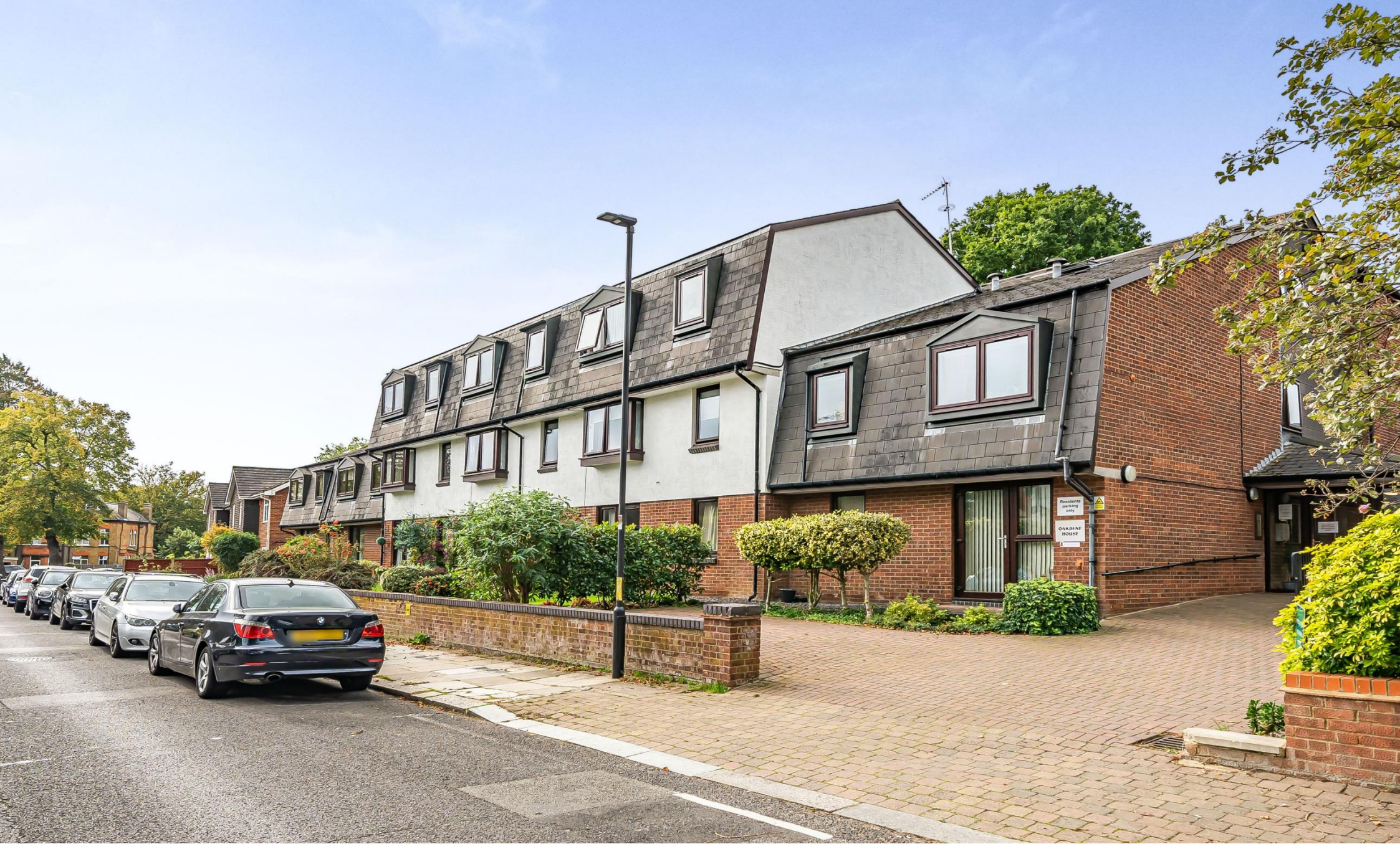
Oakdene House, Bycullah Road, Enfield, EN2 8HB
