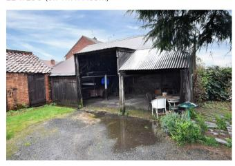
King Post Trust timber frame and corrugated tin cladding.
