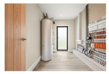
A well thought out plant room housing the main utilities with pressurised hot water system, under floor heating manifolds and electrical consumer unit, continuation of the tiled floor and obscured double glazed door into the rear garden.
