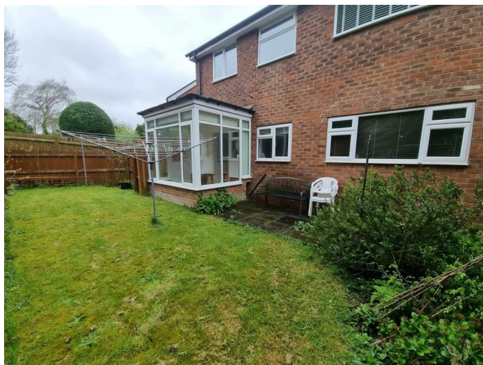
To the front we have a large fore garden mainly laid to lawn with pathway leading to front door and side access into the garden. This could easily be converted into off road parking with the relevant planning permissions.
