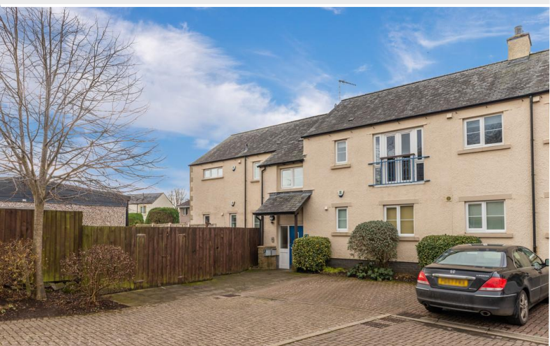
Parking Area and Communal Entrance
