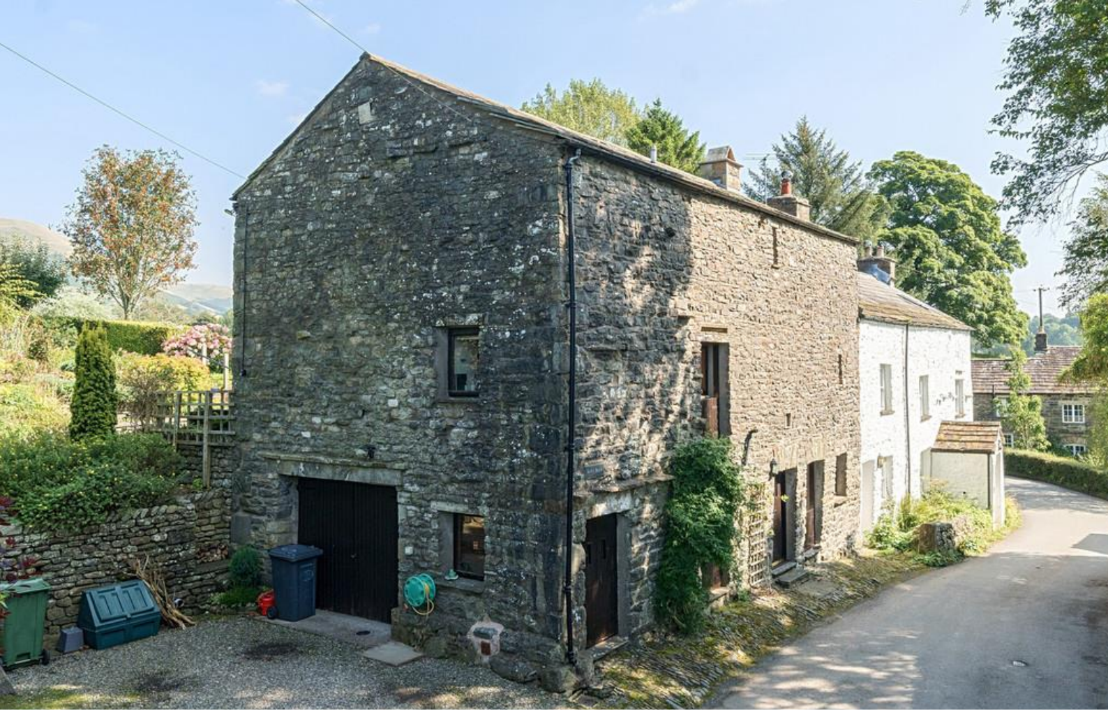
Elevated Front Aspect
