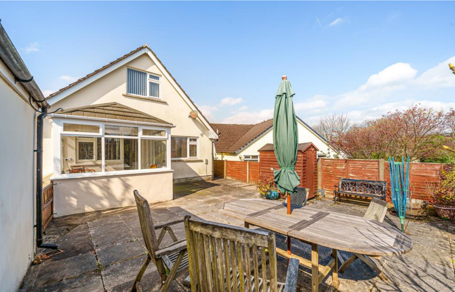
Rear Elevation & Patio Garden
