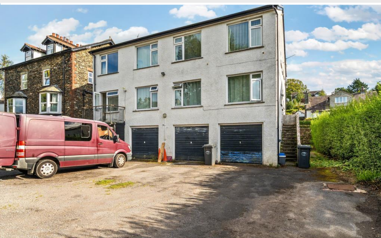
Garage and allocated parking
