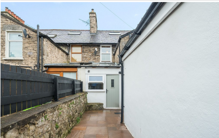
Rear Aspect and Yard
