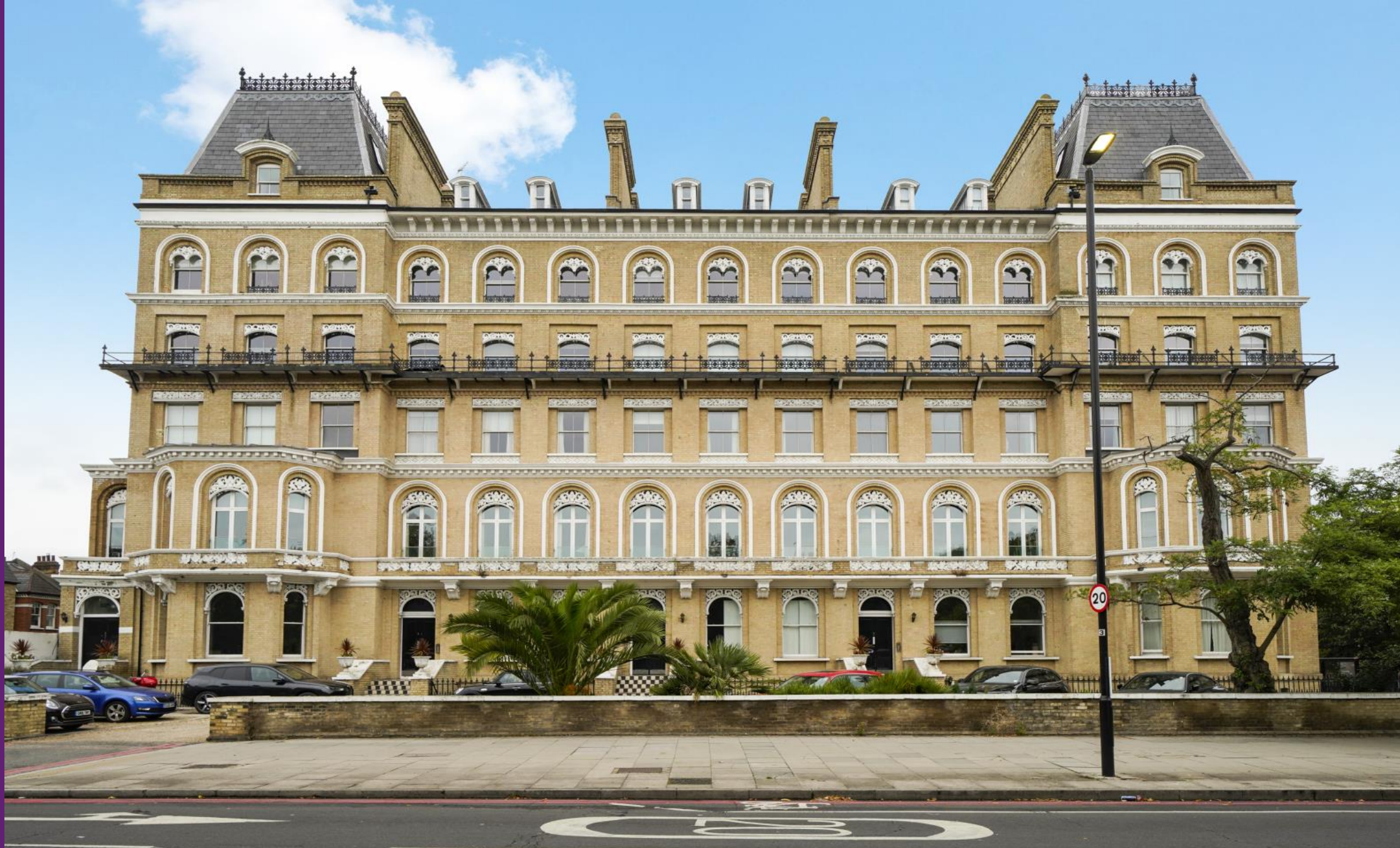
Thornton Place Clapham Common North Side, SW4
