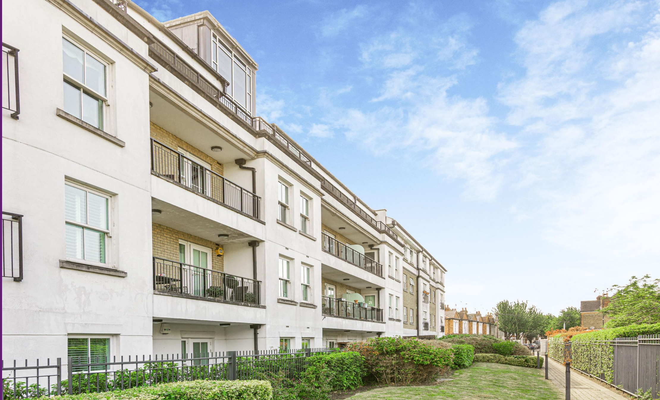
Greensward House Imperial Crescent, SW6
