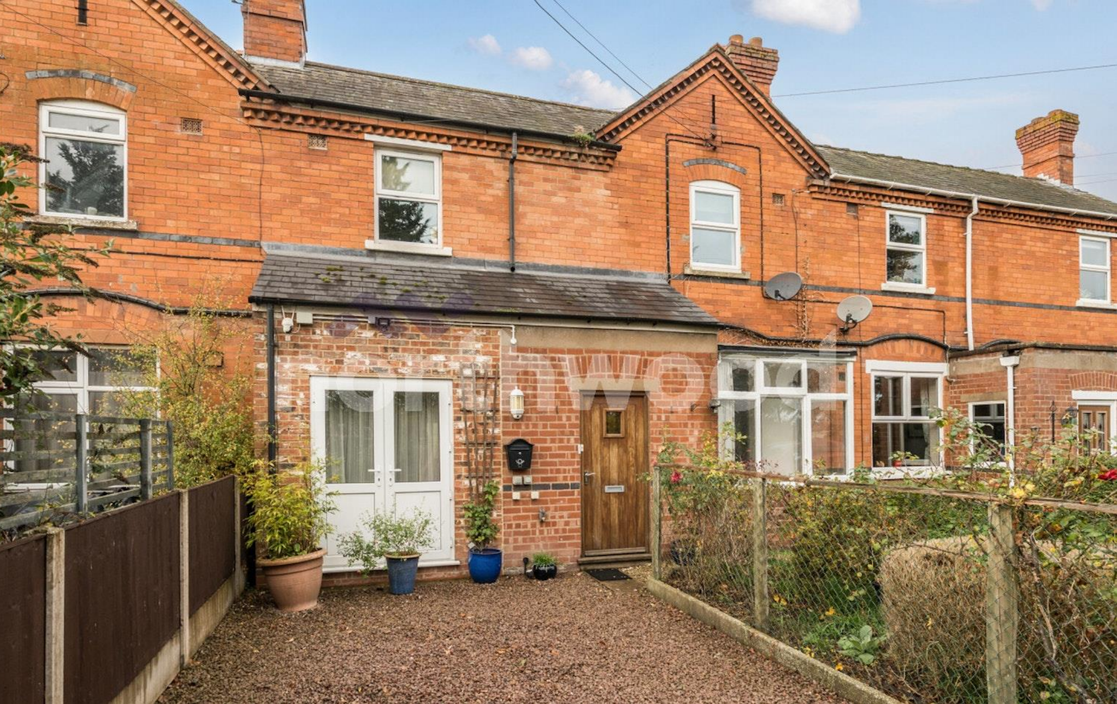
Broomhall Cottages, Worcester
