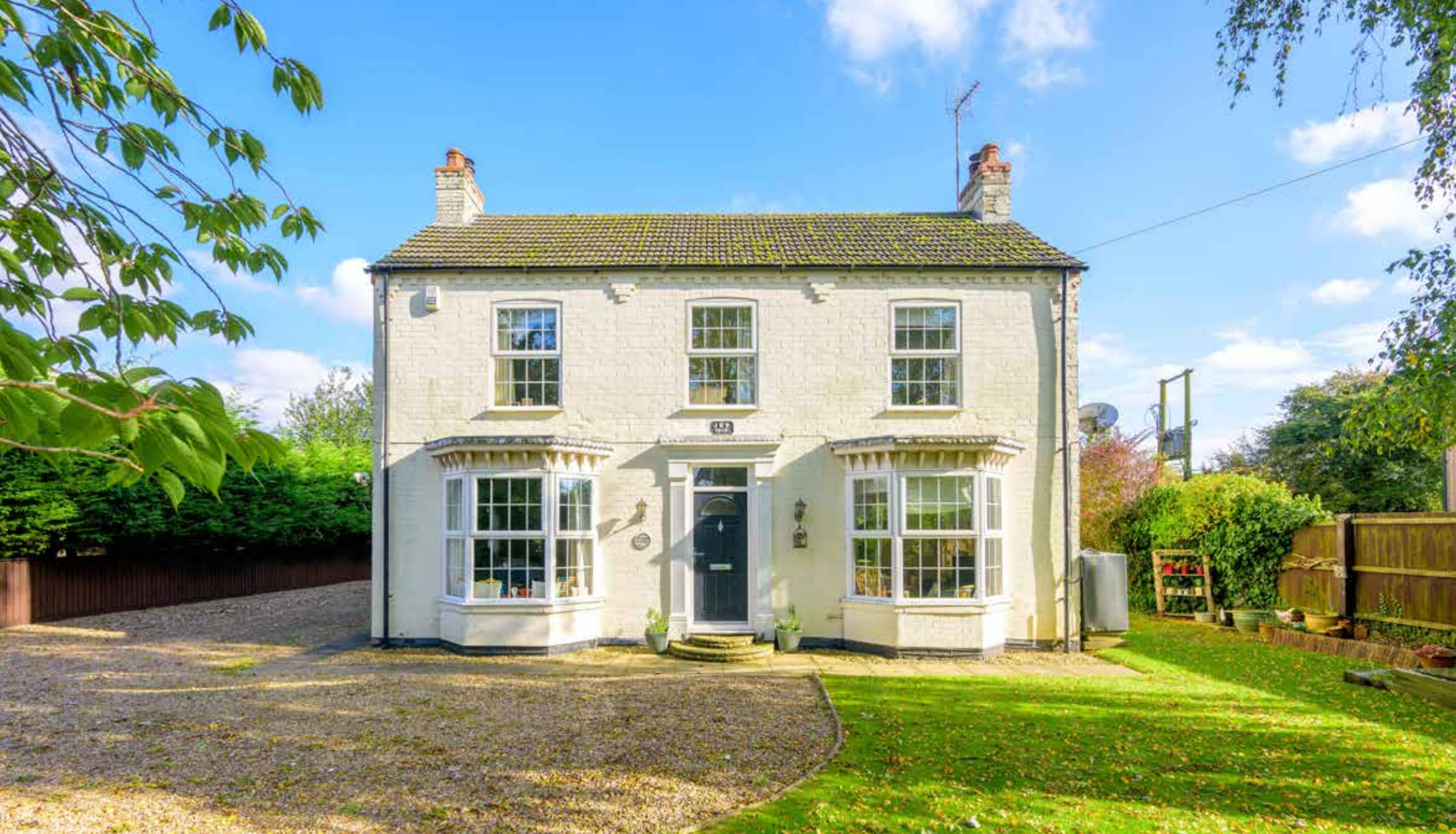
Victory House Station Road | Moulton | Lincolnshire | PE12
