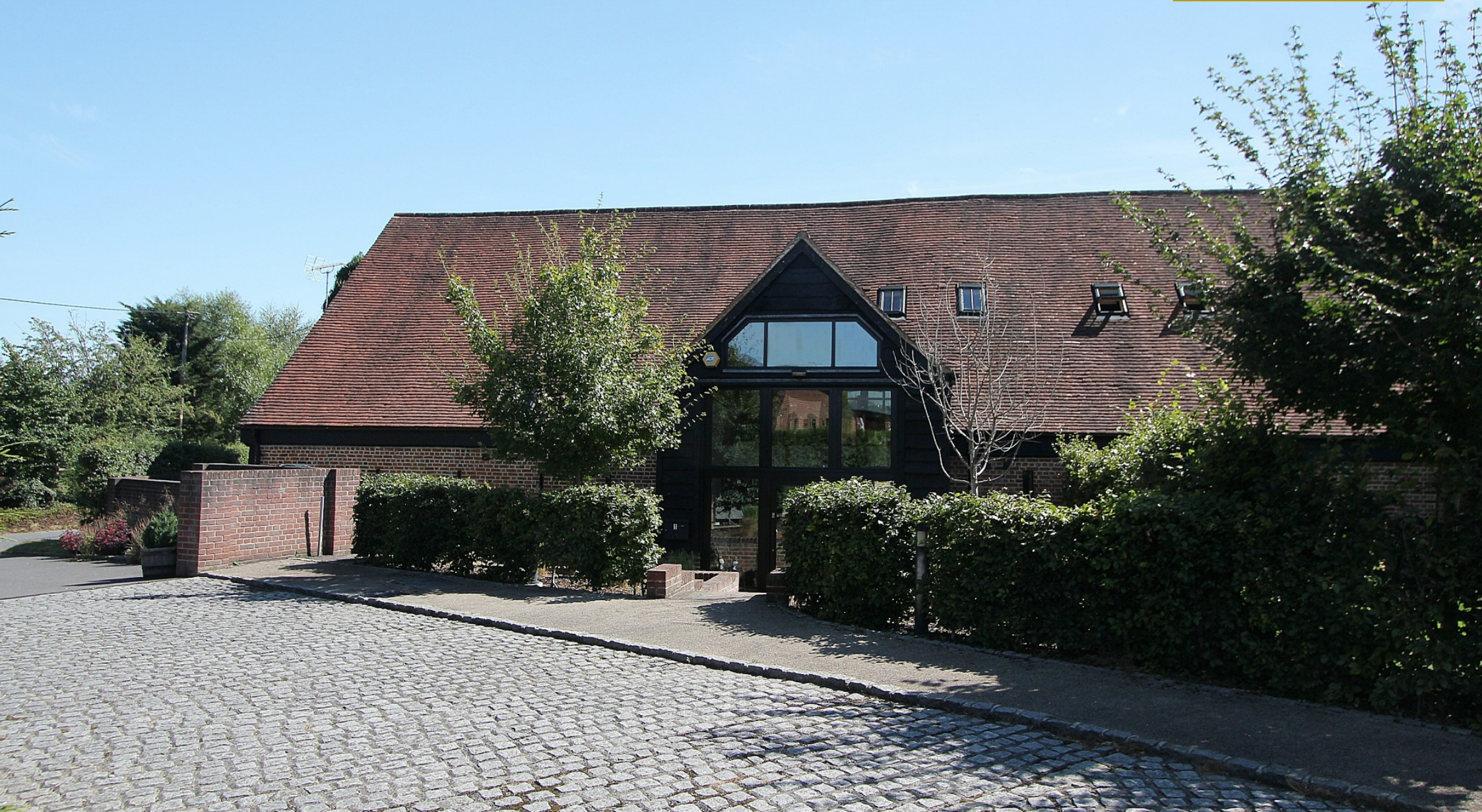
North Barn • Tidmarsh • Berkshire
