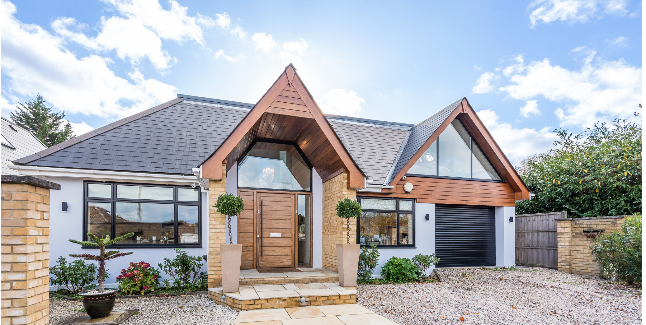
TRUMPSGREEN AVENUE, Virginia Water GU25
