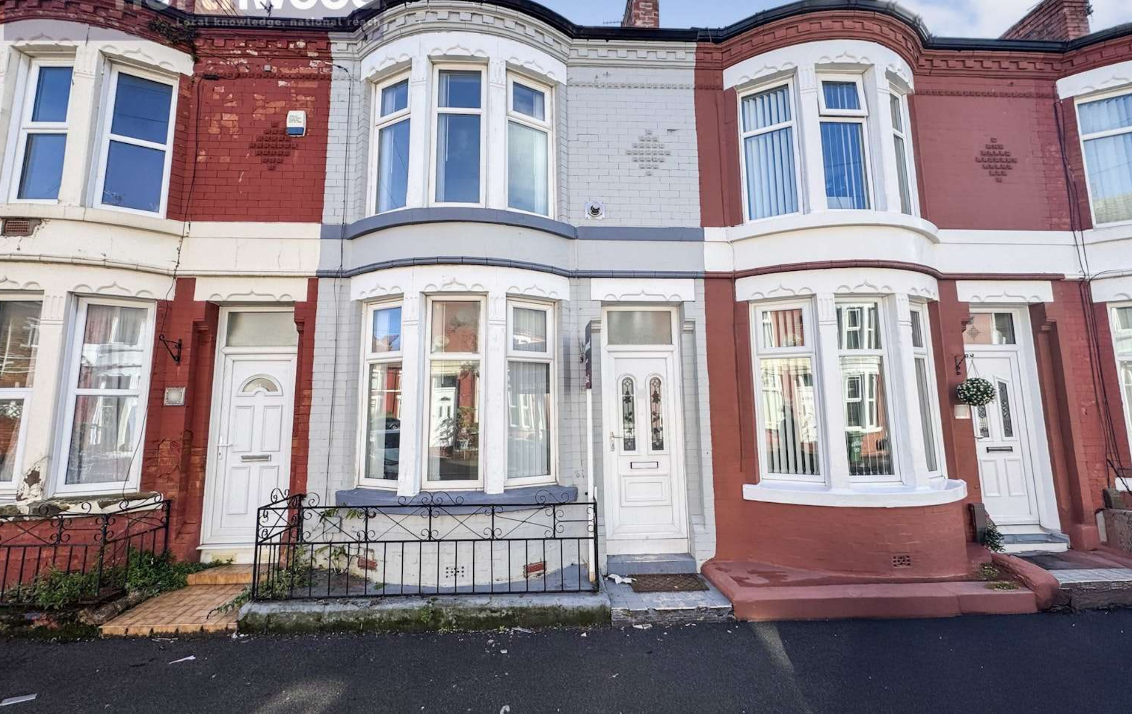
Northbrook Road, Wallasey, Wirral
