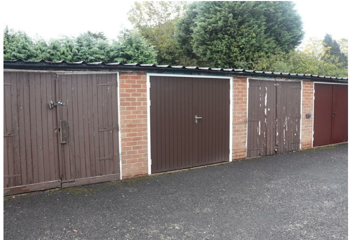
Garage in Block
