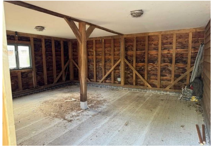
Existing Internal Space
