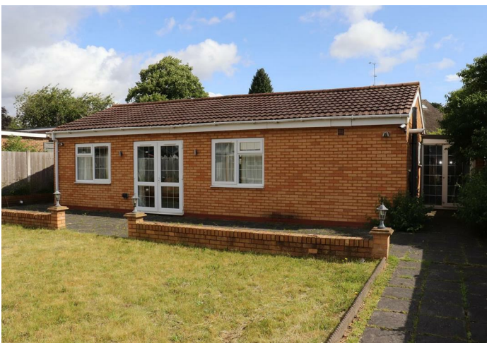
Detached Annex To Rear
