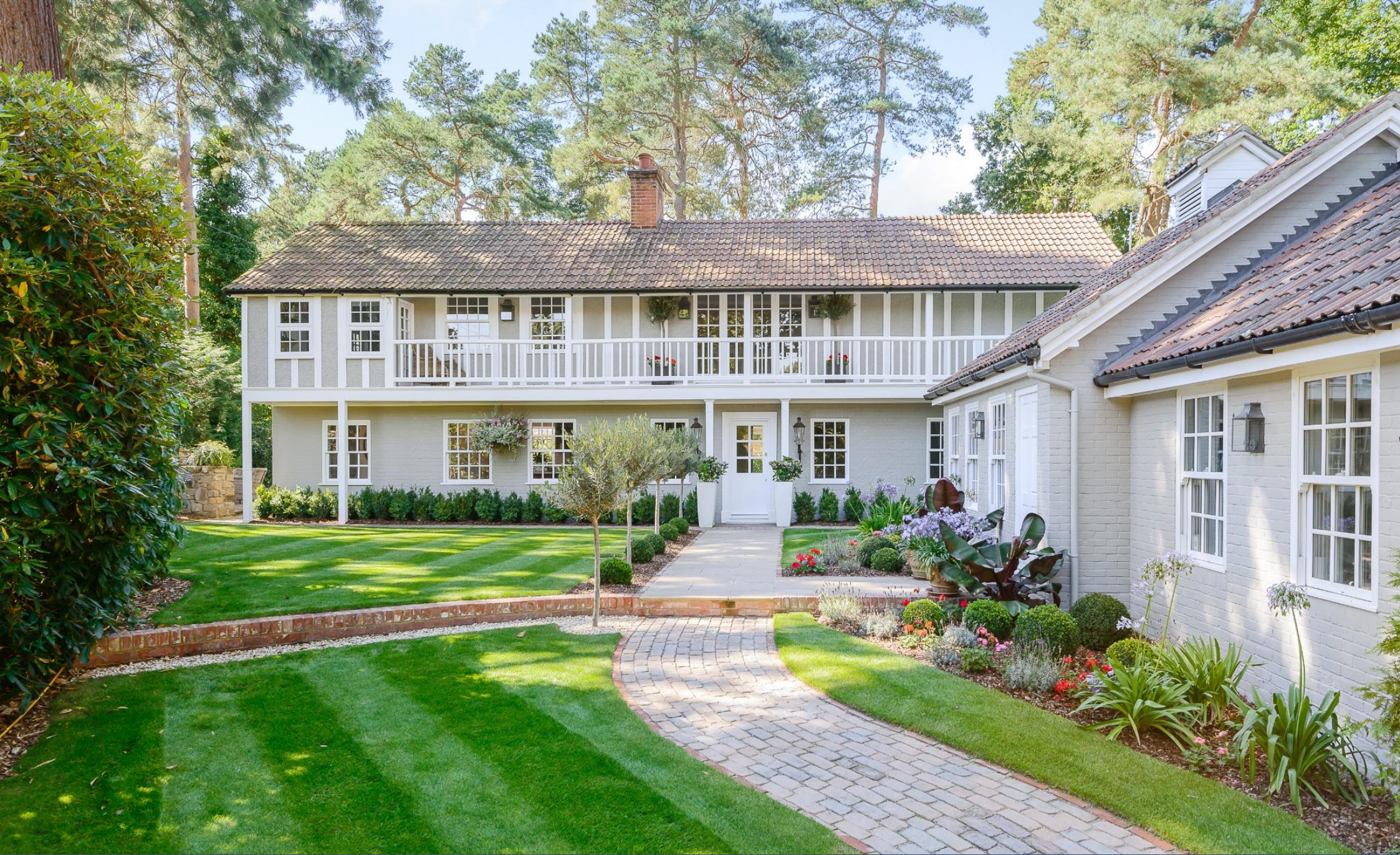
Henley House, Friary Road, Ascot
