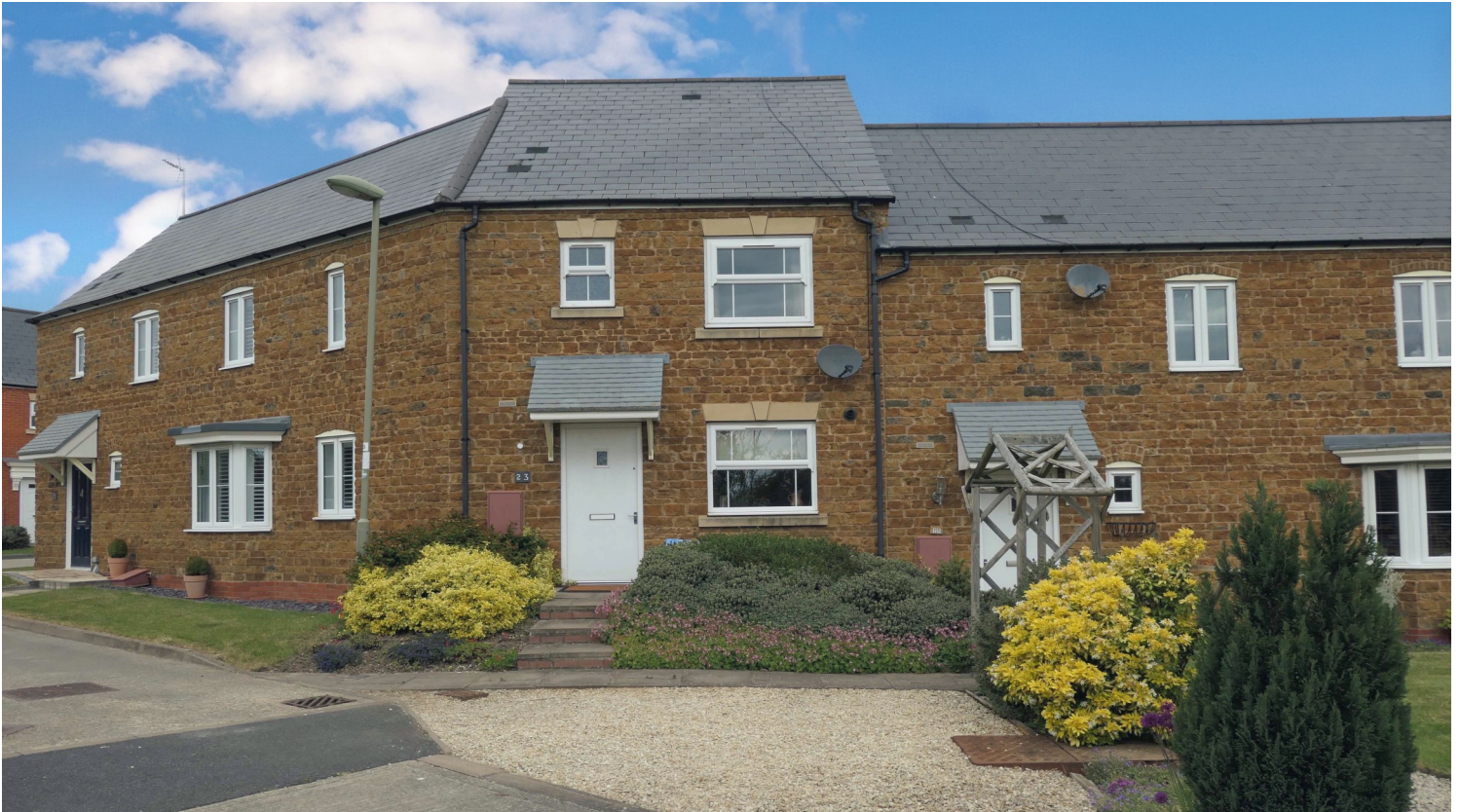
BRIDGES CLOSE, BLOXHAM, OXON, OX15 4FS
