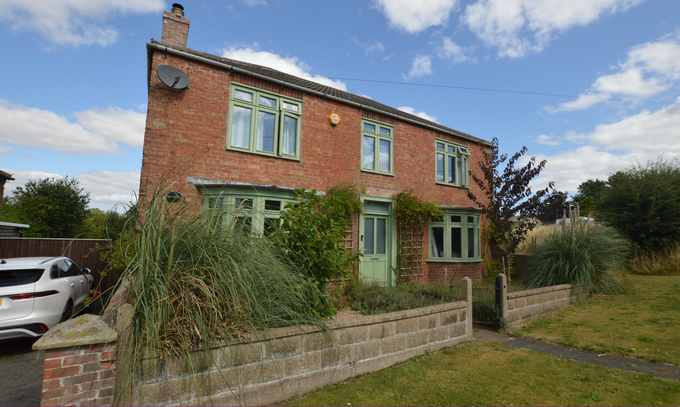
Chartwell Gainsborough Road, Glentham, LN8 2EG £389,995
