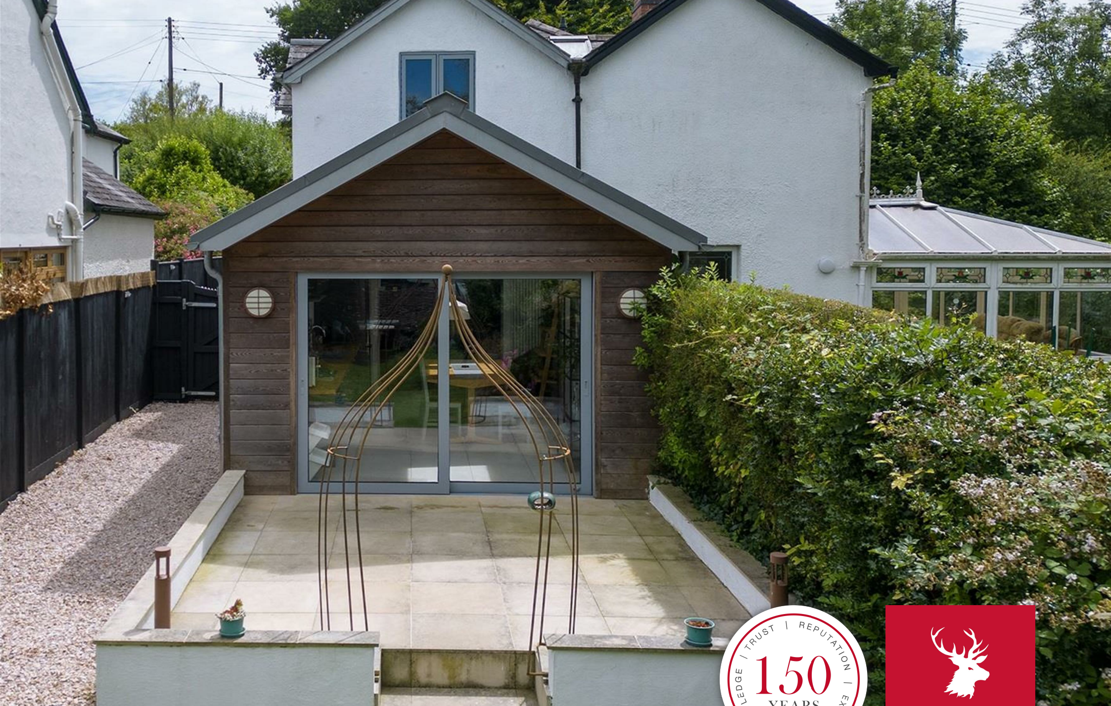
3 Bridge Cottages, Green Lane
