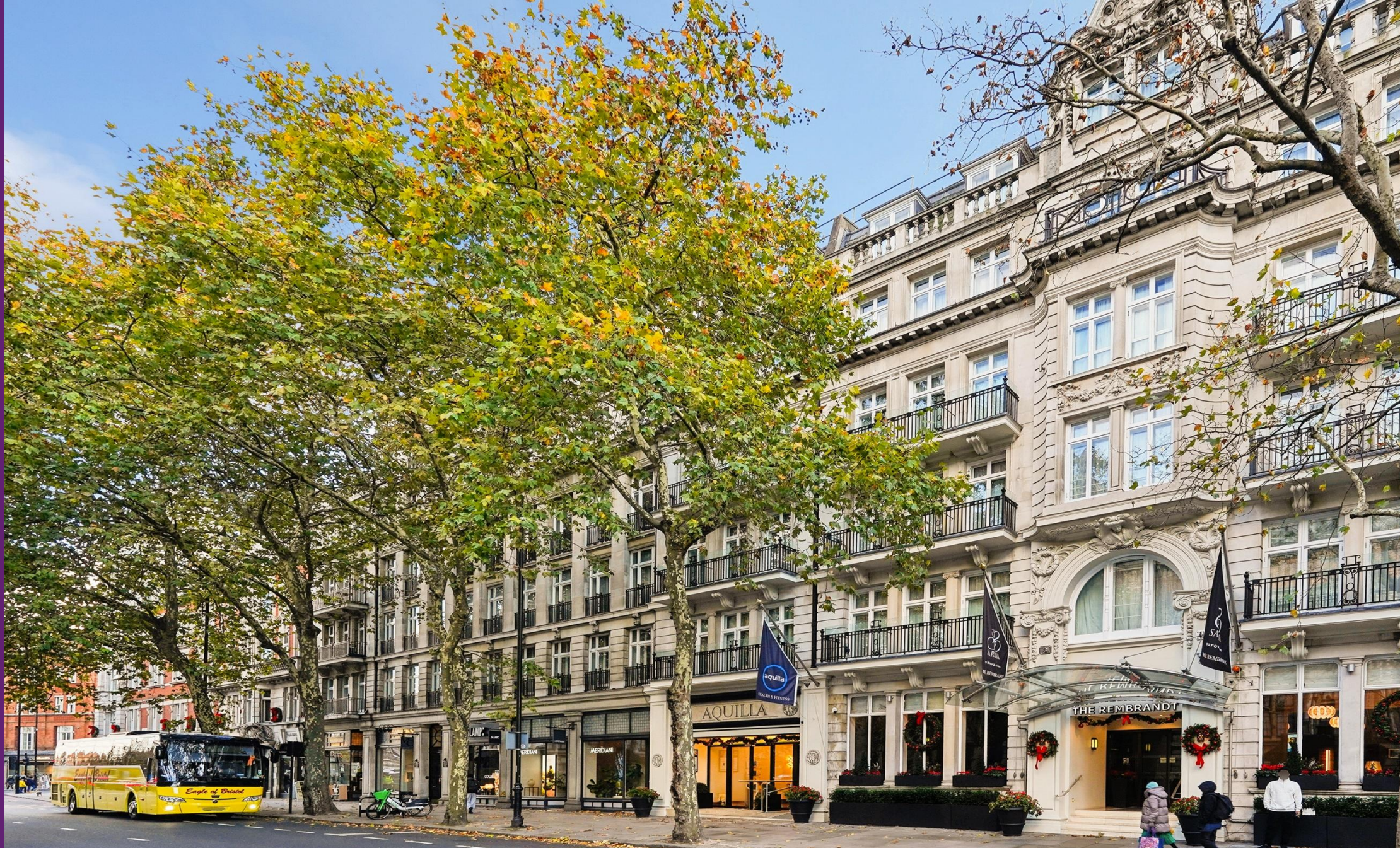
Dalmeny House South Kensington, SW7
