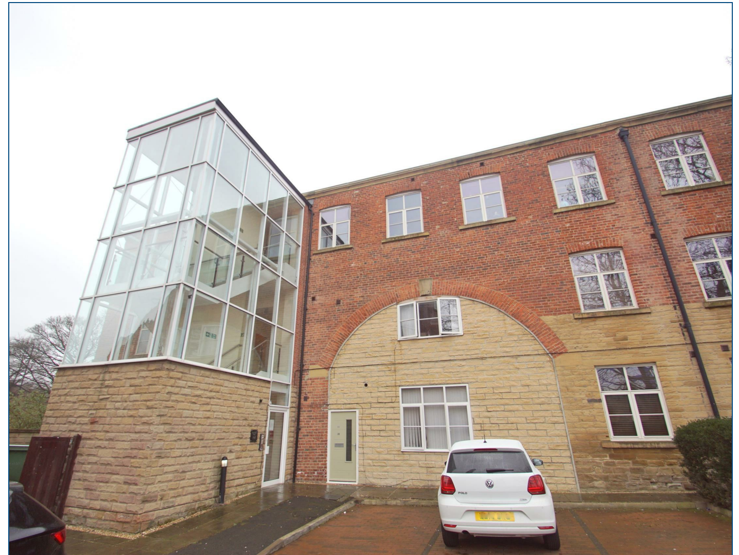
Stanningley Place, LS12 3DG
