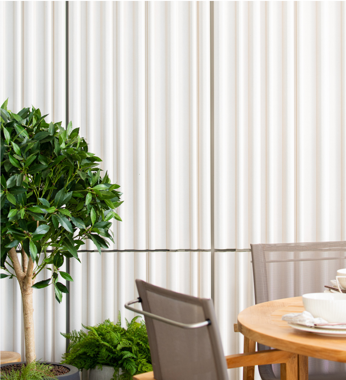
TERRACES — Floors finished with decking and fluted white terracotta cladding
