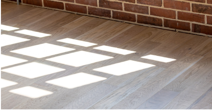
Engineered timber flooring within the apartments
