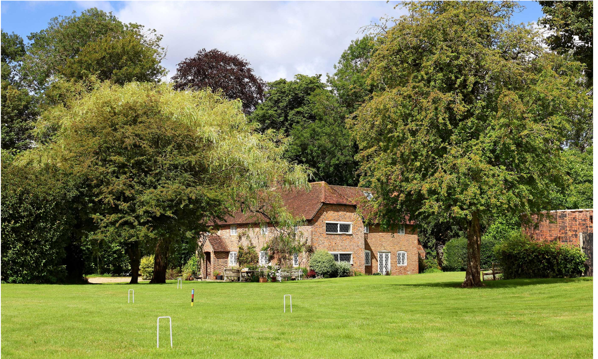
Carpenters Cottage, Burkham, Hampshire
