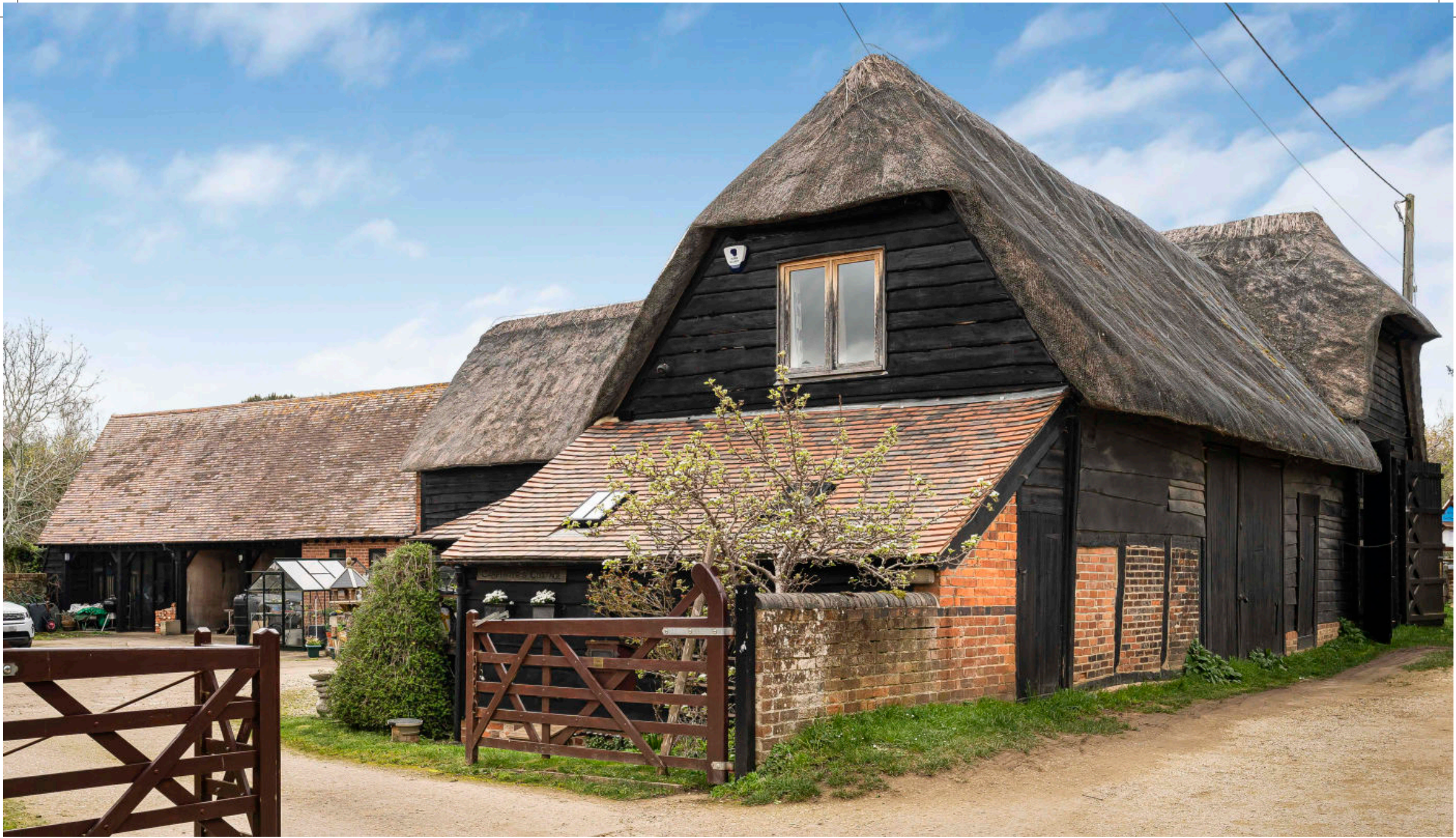
Carpenters Cottage, Long Wittenham, Abingdon
