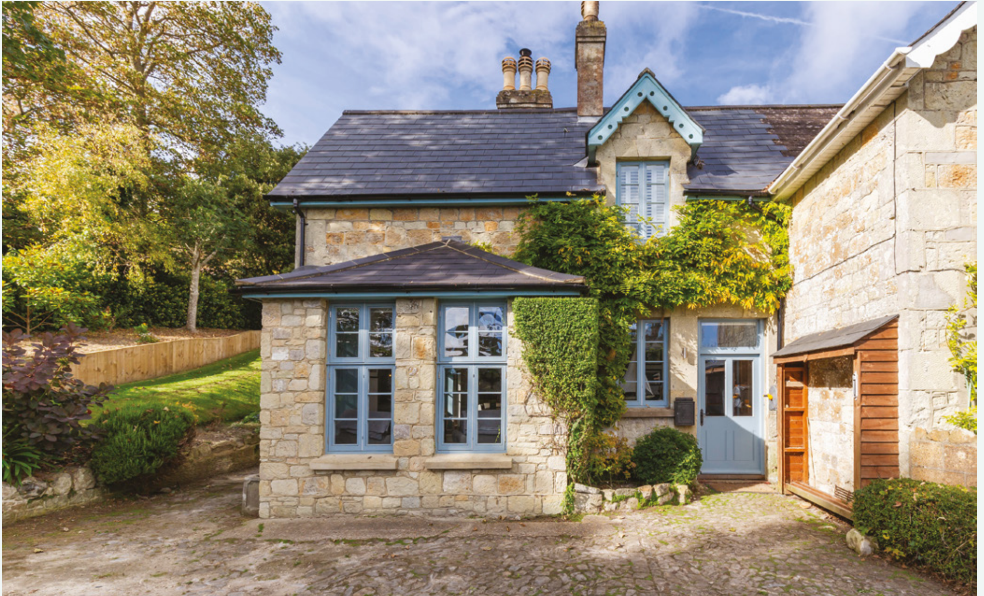
Belvedere Cottage, Old Park Road, St Lawrence, Isle of Wight
