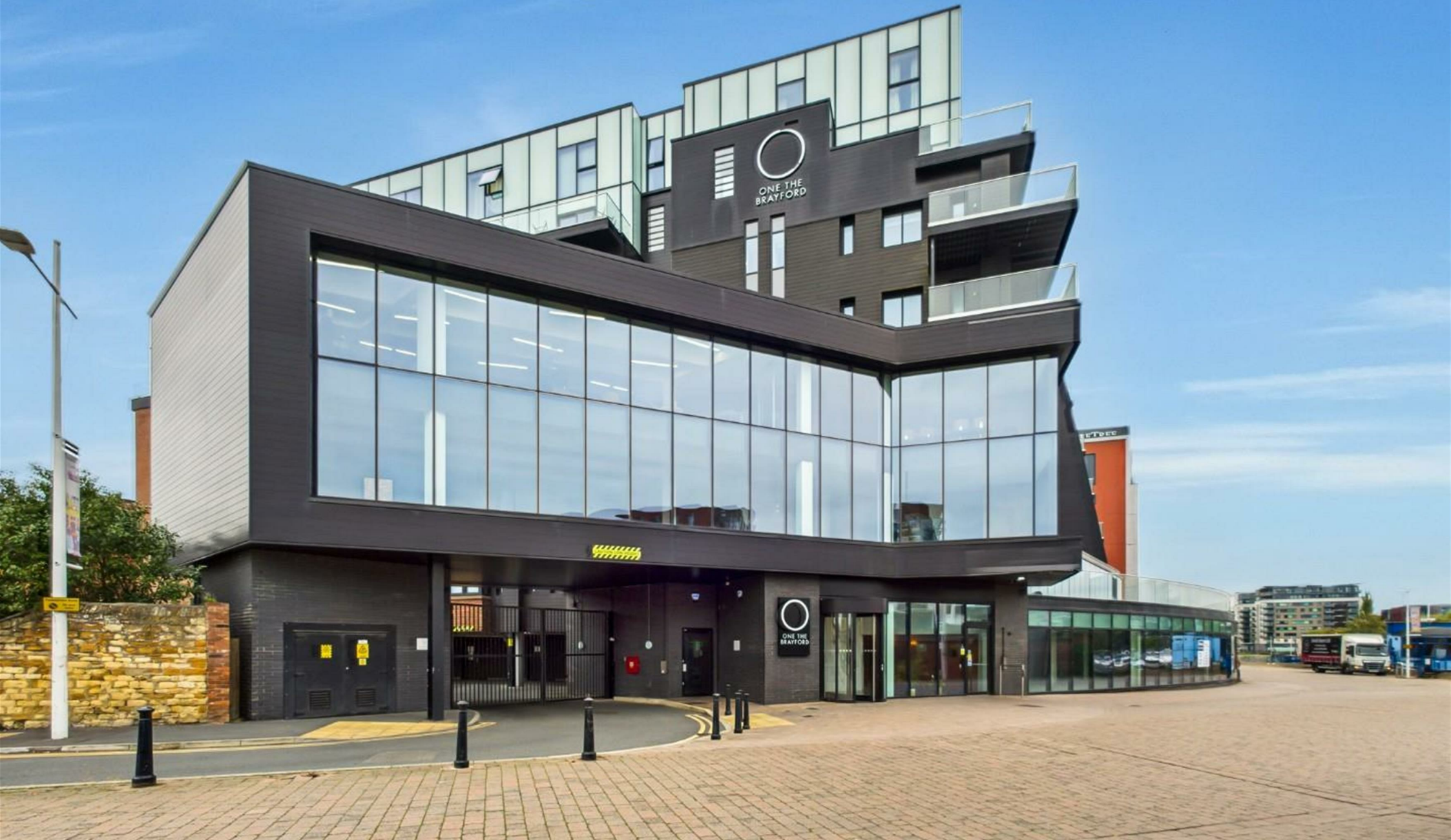
One The Brayford, Brayford Wharf North, Lincoln
