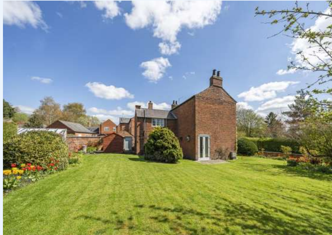
View to the front
