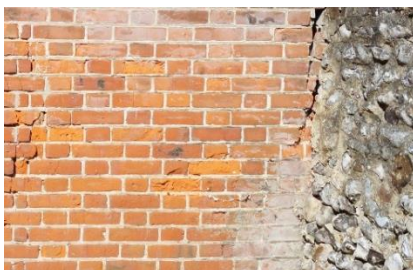
Flemish bond to garden wall: Headers and stretchers alternate in each course, with staggered joints
